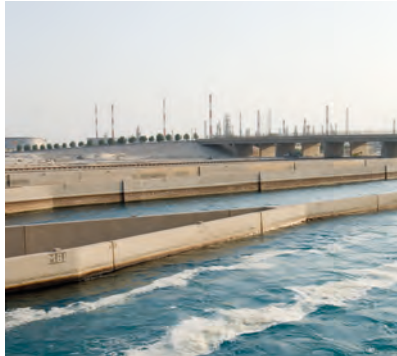
The Jubail plant uses a seawater cooling system.
